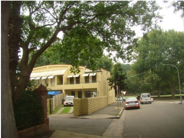
Figure 24. Rear of 2A-2D Wentworth Park Road showing slight elevation, view looking north.
