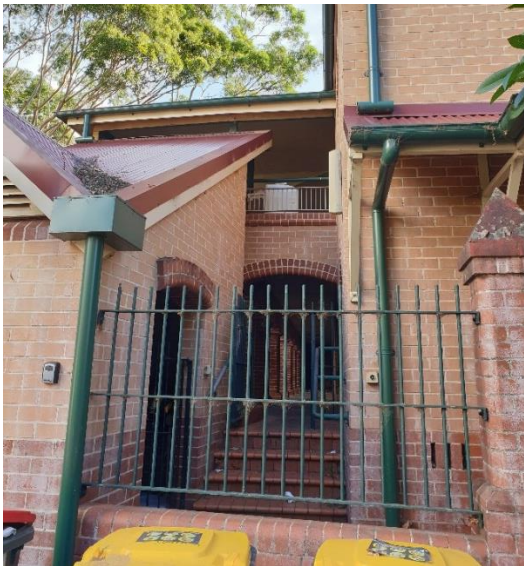
Figure 26. Stairwell at the north access to central courtyard of 17-31 Cowper Street, view looking south.
