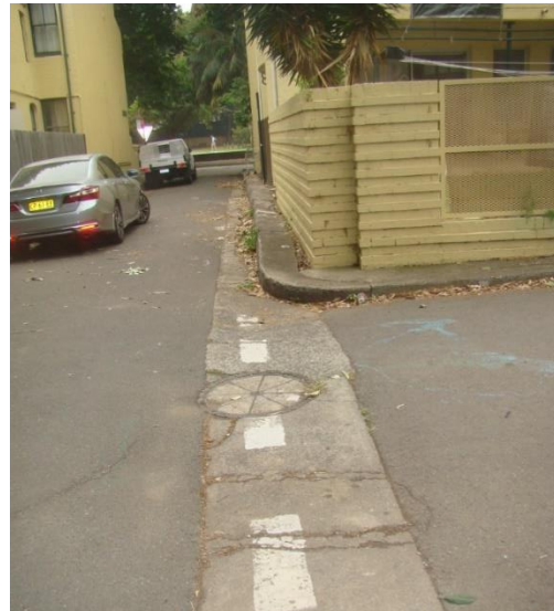
Figure 27. Services along Mitchell Lane, looking north.
